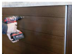
2. Unscrew and remove cabinet panel.
